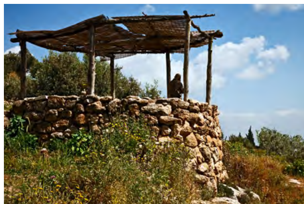
A tower in a Nazareth village in Israel, like the tower described in Luke 14:28–30
